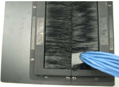
Figure 4. The position of cable bundles in brush-style grommets can move bristles out of position to reduce sealing effectiveness. In addition, bristles can sag, degrade, or break off over time.
